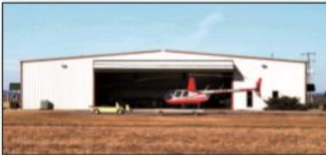
All buildings at Stigler Regional Airport are designed to sustain 100-mile-per-hour winds.
